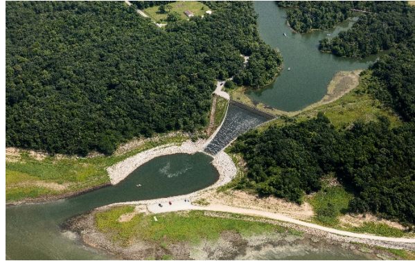
Big Creek Diversion Channel & Terminal Dam/Spillway with water flow into Saylorville Lake
