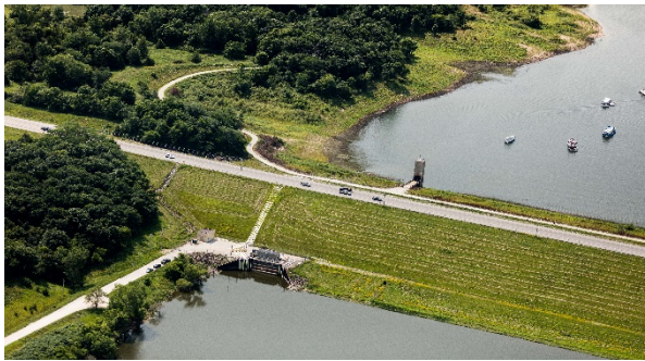
Big Creek Barrier Dam & Pump Station
